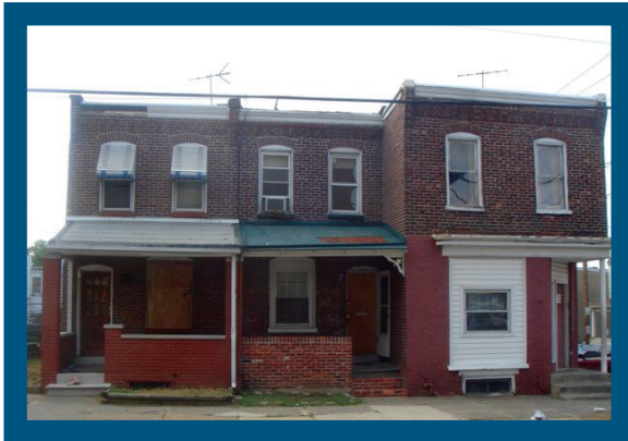
DuPont Street housing unit prior to renovation
